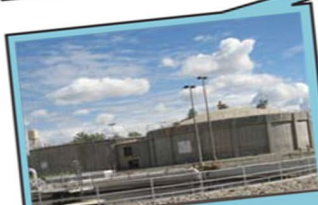
Digesters Microorganisms kept at 98 degrees F produce methane gas.
