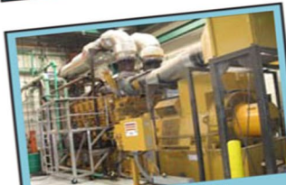
CoGen Facility (Generator) Methane gas is burned to create electricity that runs our plant.
