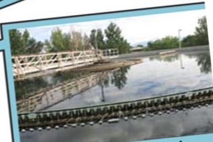
Secondary Clarification Tank Fat, old microorganisms settle out and activated sludge is sent to aeration.
