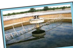
Primary Clarification Tank Sludge settles out at the bottom while grease is skimmed off the top.
