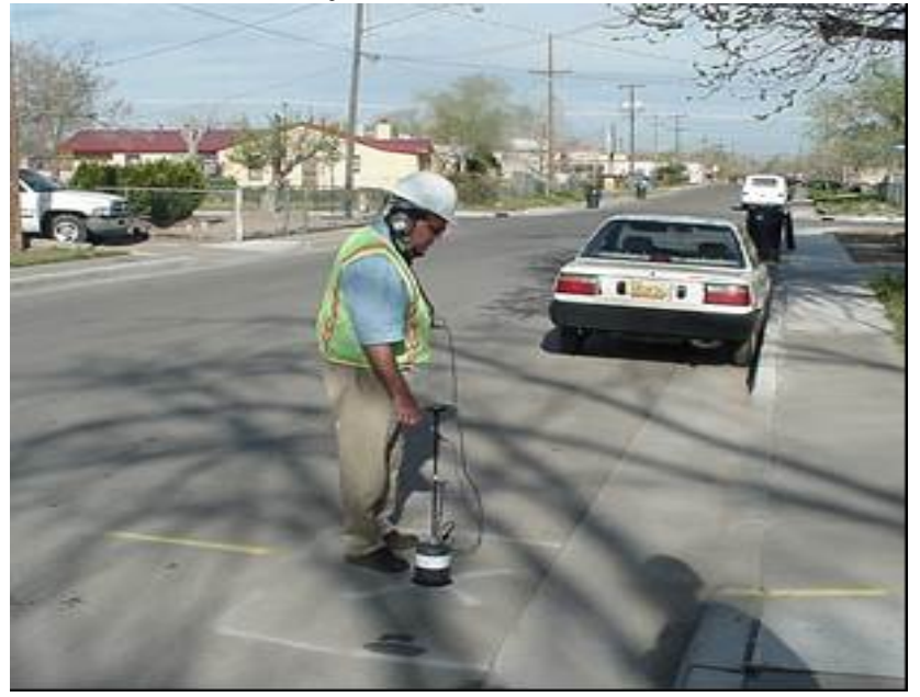
Leak Detection Survey
