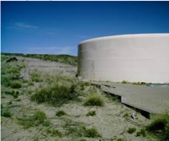
Existing College Reservoir No. 1
