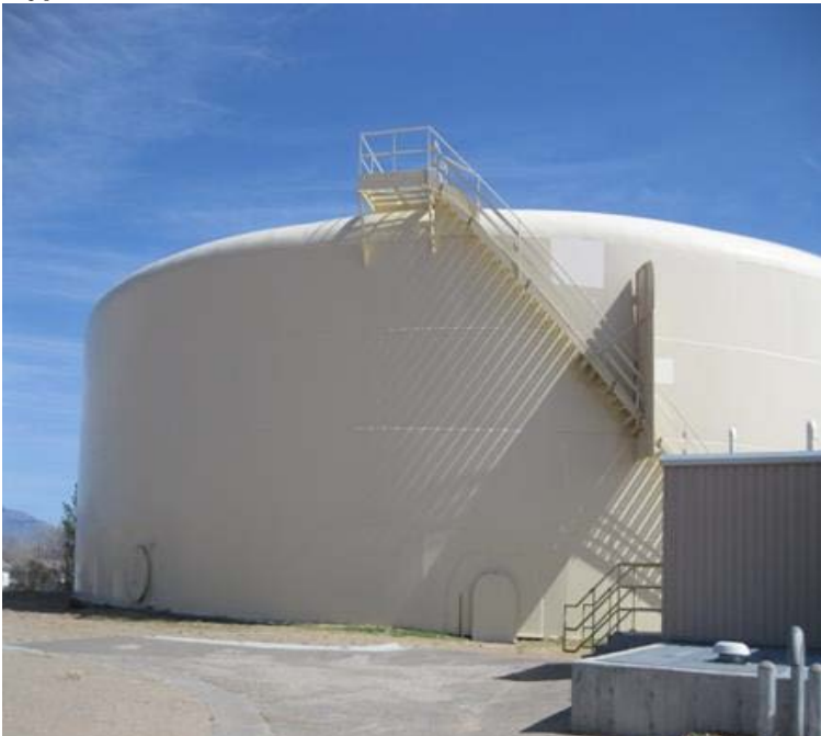
Typical Potable Water Reservoir
