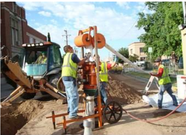
8-inch Sewer Lining Installation Project Downtown at 7th Street and Kent
