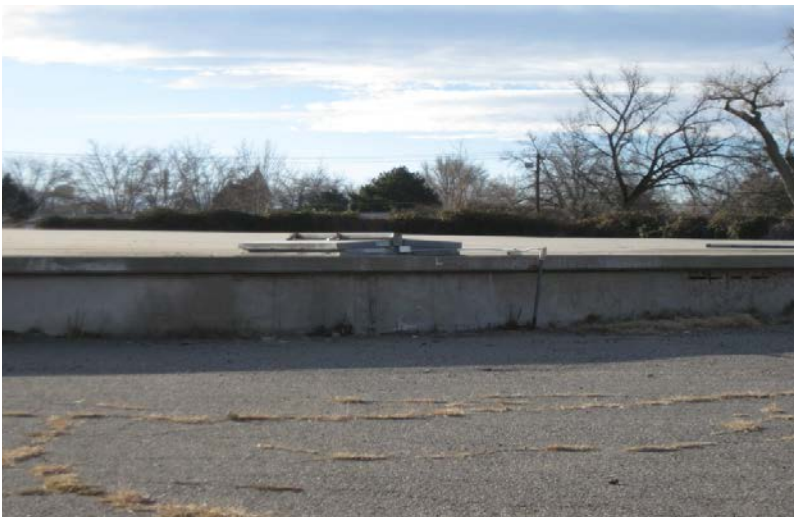
Charles Wells Reservoir - Concrete Tank
