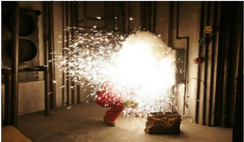
Arc flash engulfing a worker
