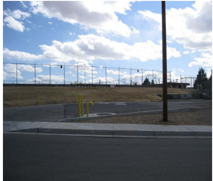
Charles Wells Reservoir from Street
