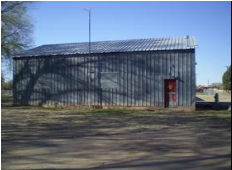
Griegos Pump Station - Exterior
