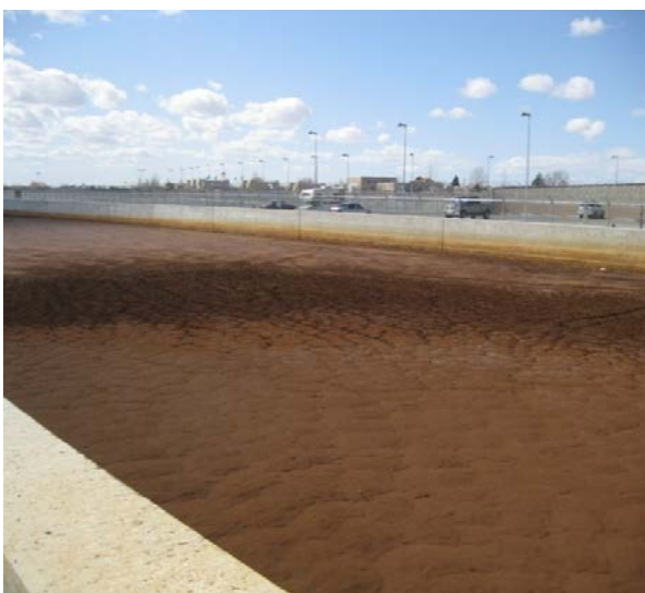
Sludge Drying Bed at SJCWTP
