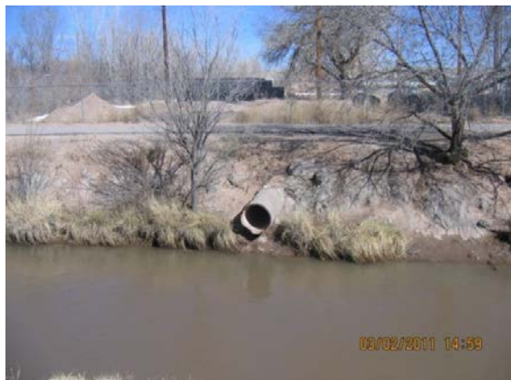
One of 3 storm water discharge points from SWRP
