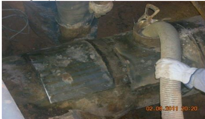
Patching the pipe with a welded plate
