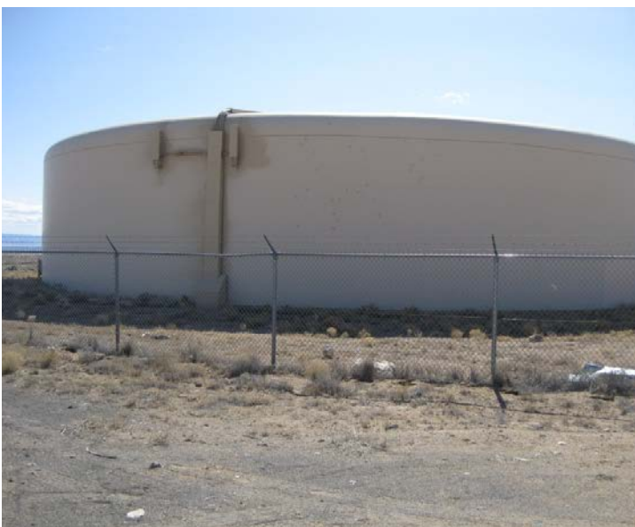
Corrales Reservoir No. 6
