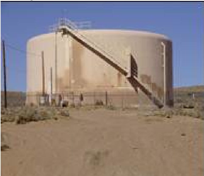
Existing Franciscan Reservoir
