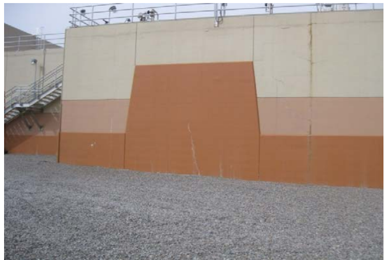
Relocate Monitoring Stations to Side of Contactor Basins
