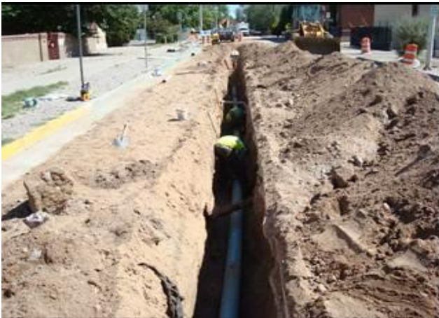
New 6-inch Water Line Installation
