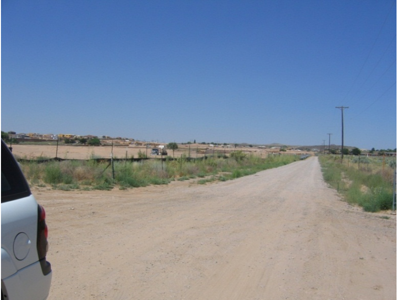
Lift Station #24 adjacent to new development
