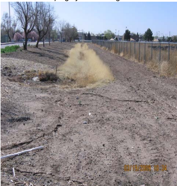
Failed Landscaping by Dewatering
