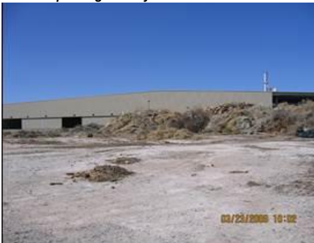
SAF Composting Facility
