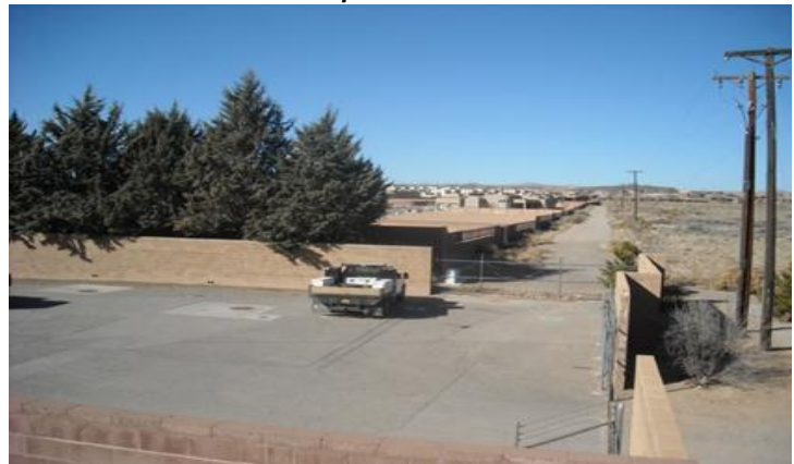
Lift Station #24 with development next to station
