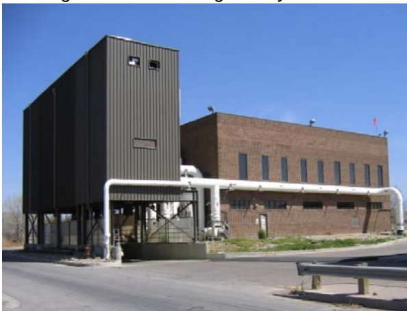
Existing Solids Dewatering Facility
