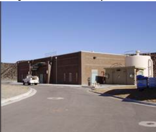
College Arsenic Removal Facility
