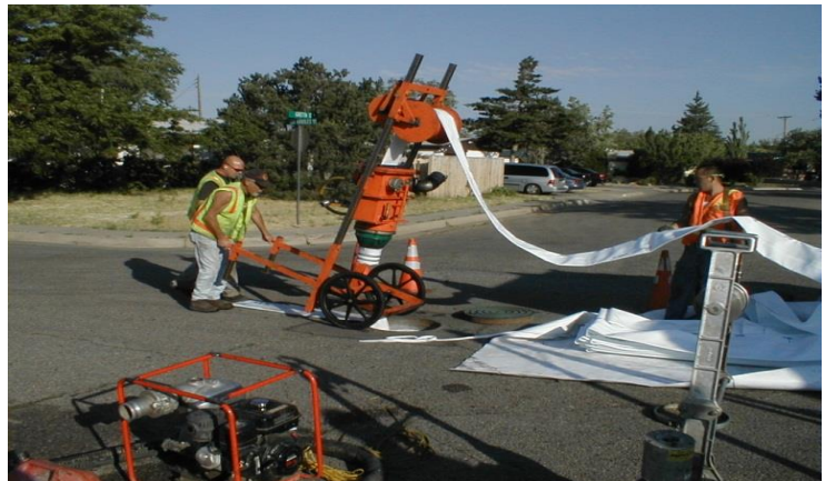
8-inch Sewer Lining Project on Los Arboles NE
