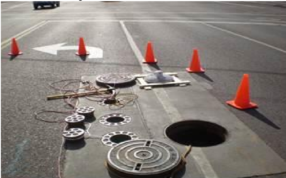
New Pressure Reducing Valve installation
