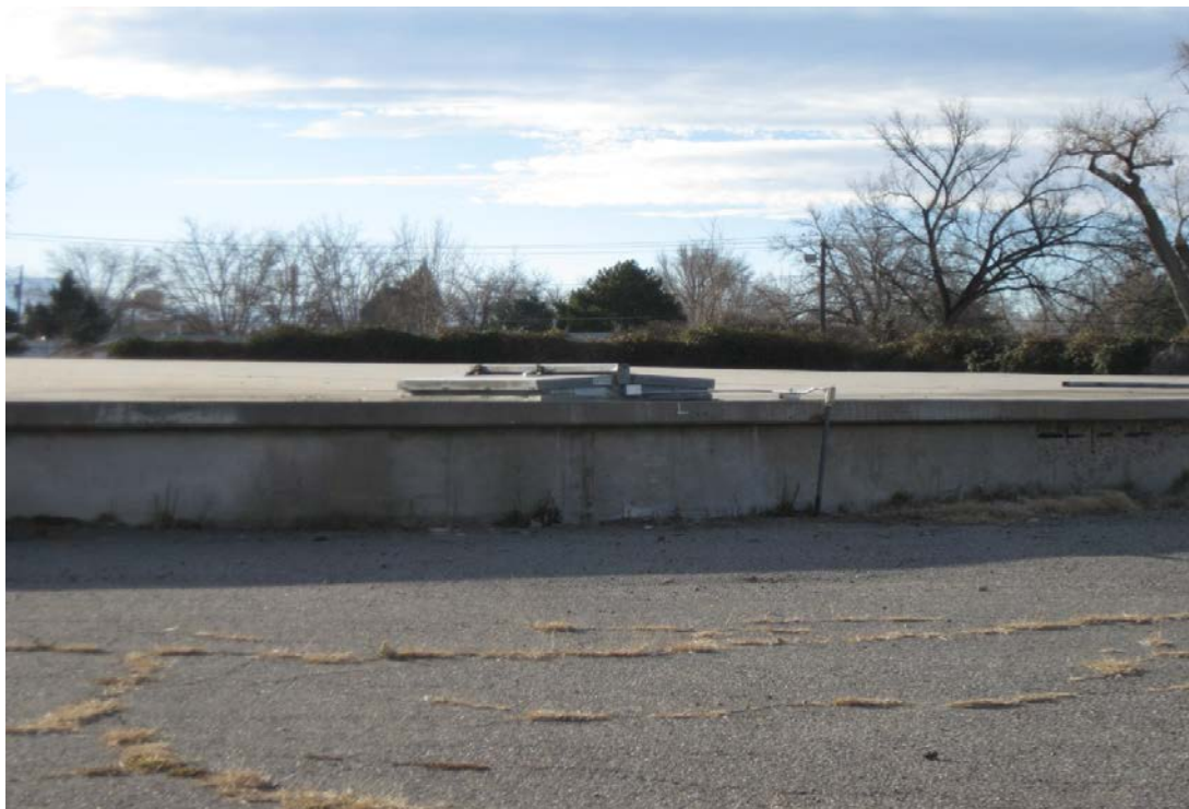
Burton Reservoir No. 2 - Roof Hatch
