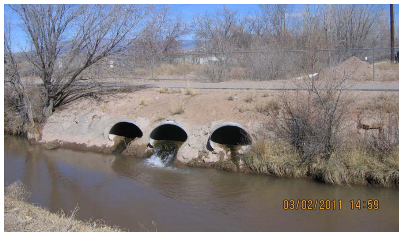
Main SWRP storm water outfall; Discharge is from construction ground water control
