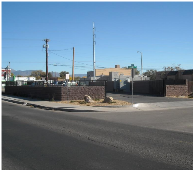
Odor Control Station 51. 2nd St. & Griegos
