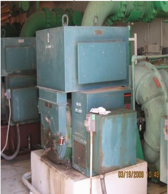
A Hoffman multi-stage centrifugal blower
