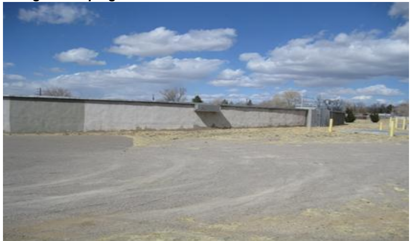
Griegos Pumping Station
