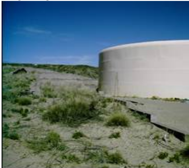
Existing College Reservoir No. 1
