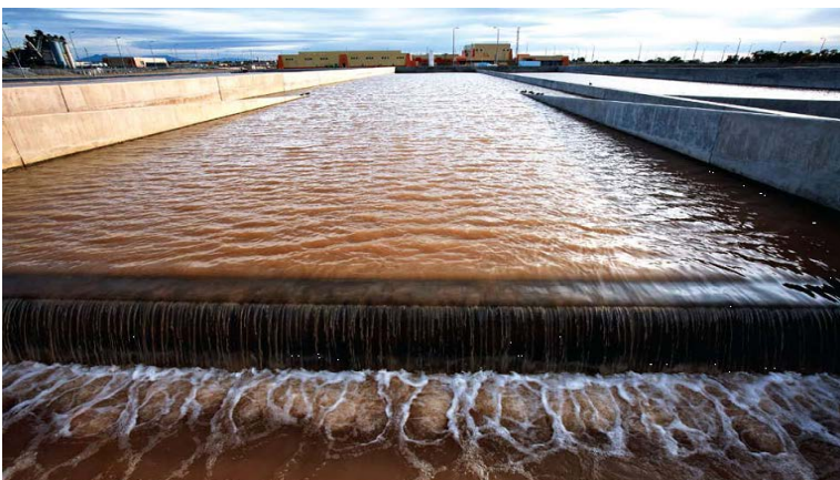
Grit Removal Basin at the SJCWTP
