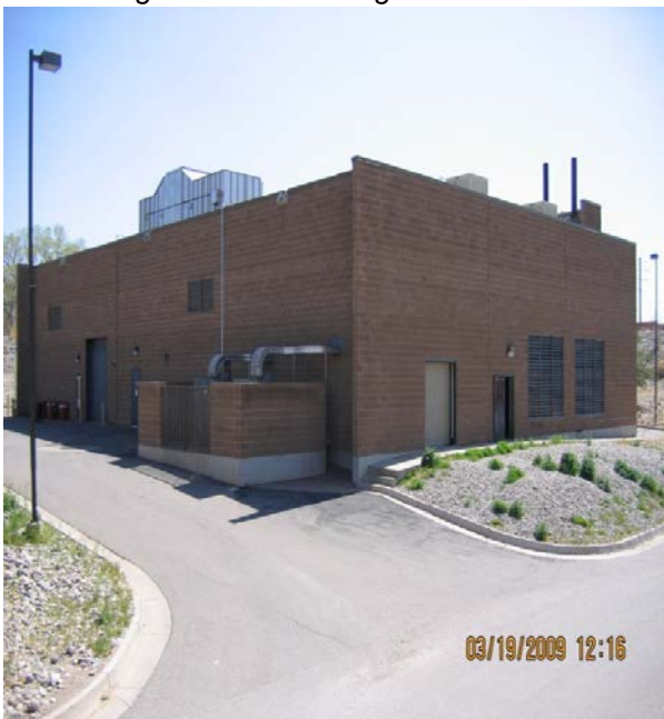
South Cogeneration Building
