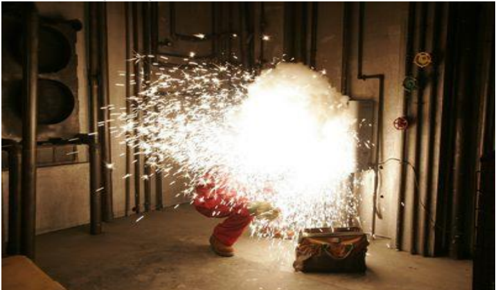
Arc flash engulfing a worker
