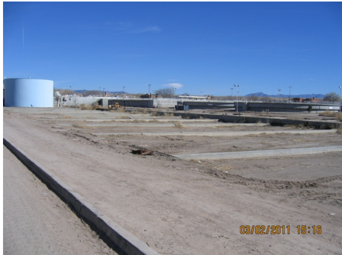
View of original sludge drying beds looking south
