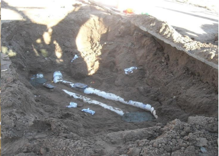
Force Main Repair - Station 68
