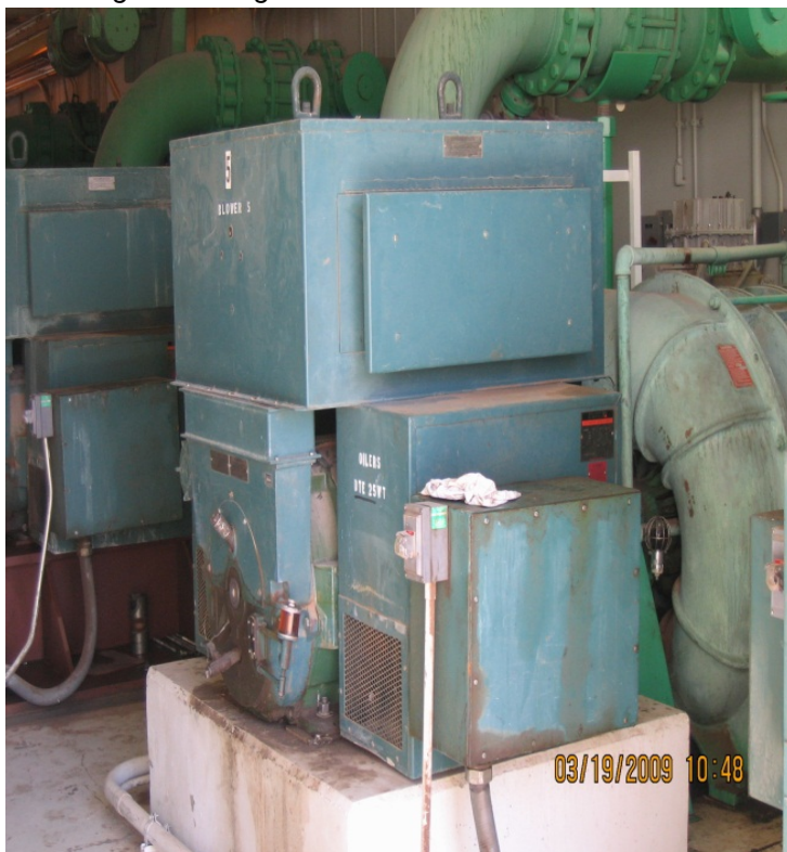
Multi-Stage Centrifugal Blower
