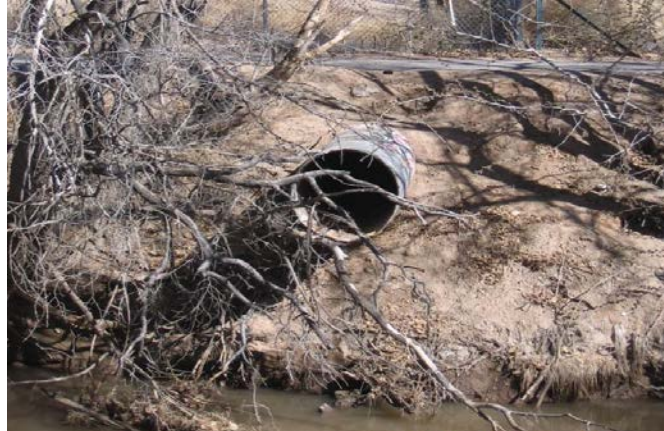
Main SWRP storm water outfall; Discharge is from construction ground water control
