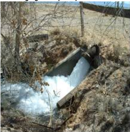
Discharging into Open Space
