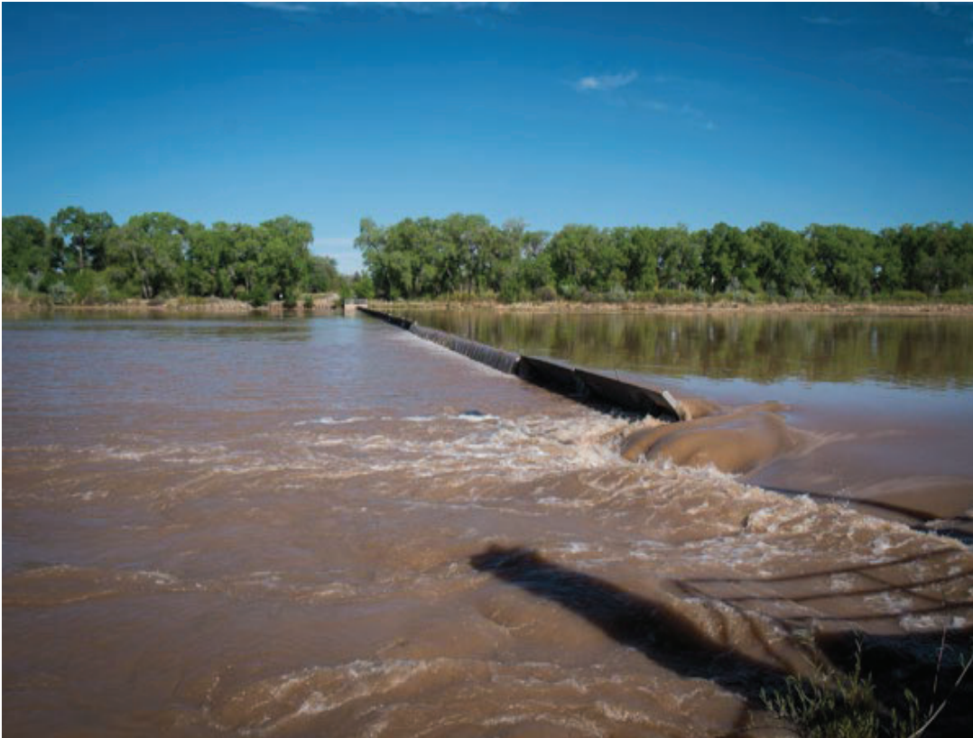
Diversion Dam off the Rio Grande River
