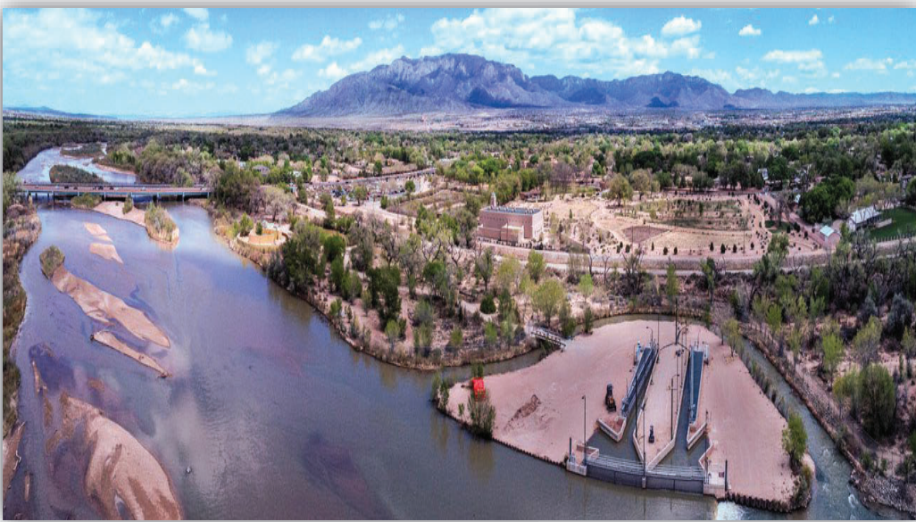
*San Juan-Chama Water Treatment Plant - Raw Water Diversion Channel
