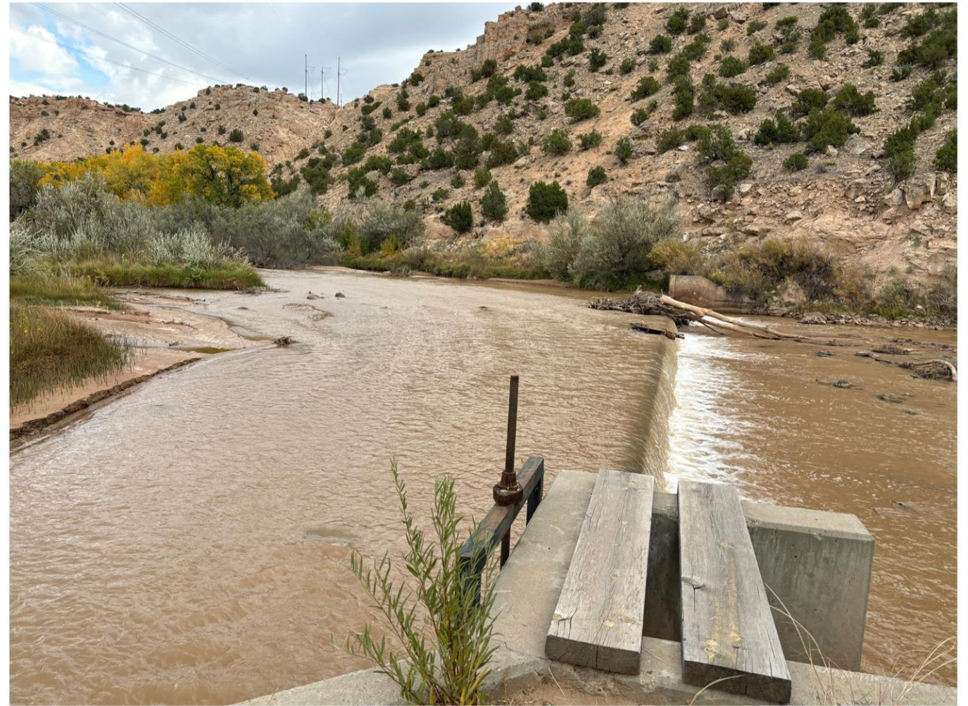
Photo: Chili Diversion (taken 10/17/2024)
