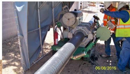
Fusing Double-Walled Groundwater Pipeline
