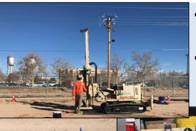
Eight SVMWs were placed at areas that are most likely to allow migration of soil vapor (utility corridors) or accumulate soil vapor (beneath pavement)
