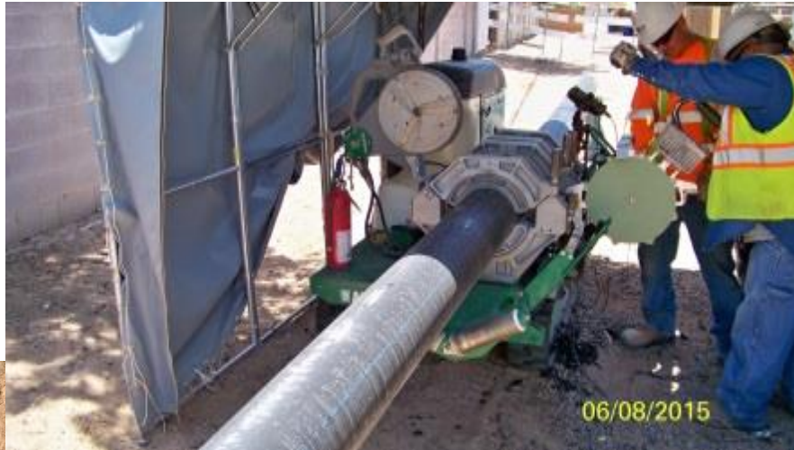
Fusing Double-Walled Groundwater Pipeline
