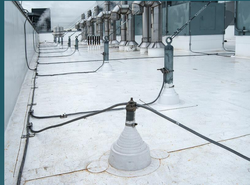
Improve Grounding of structures and connect to rooftop air terminals
