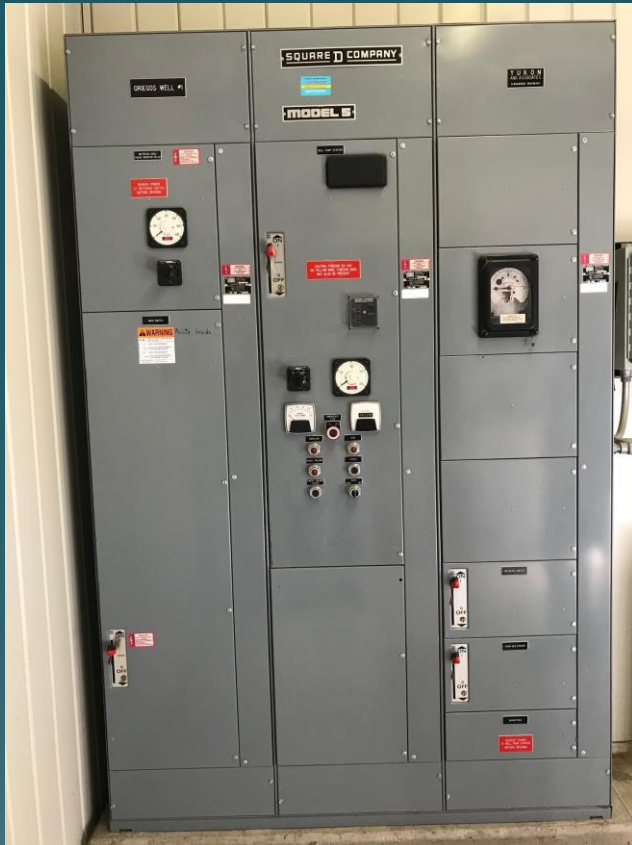
Antiquated & undersized motor control center
