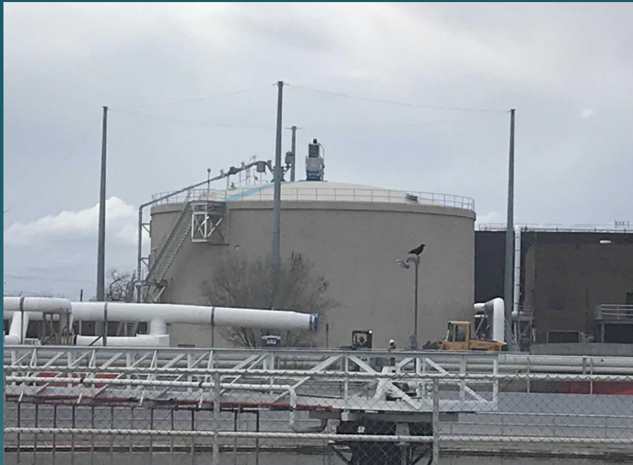
Catenary System to protect Digesters and Gas Holders
