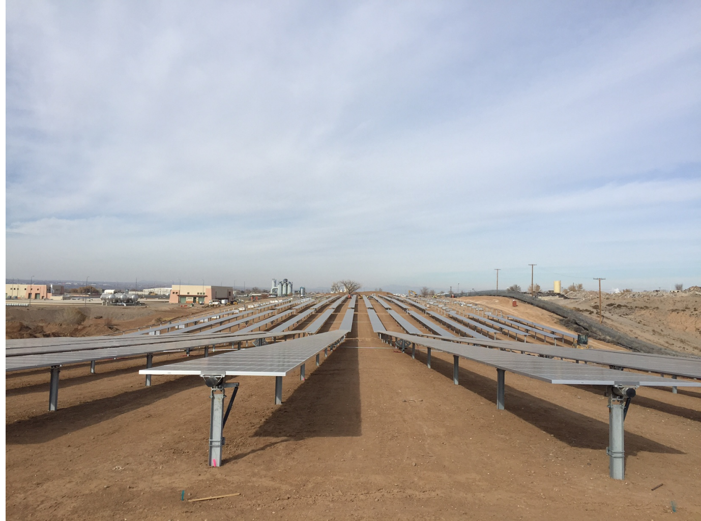
1.9MW single axis tracking array
